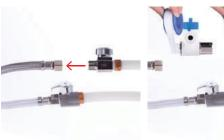
2. Detach the cold waterline from the cold water valve.
