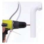
1. Choose where the drain clamp will be installed and drill a ¼inch. hole. The foam padding to the inside of the Drain clamp, around the hole.
